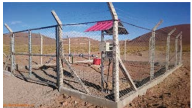
Water well number 6 of Jalanta—San Cristóbal.
